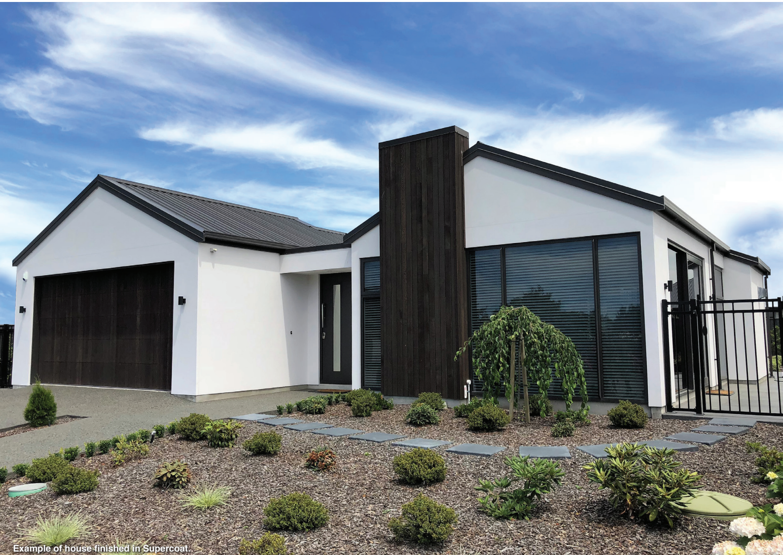
Example of house finished in Supercoat
